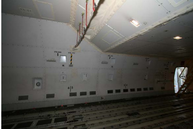
Picture 1 Cargo Compartment Liner Transition Panels At The Fire Location
